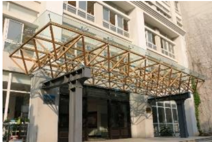
Fig.8. Steel and glulam hybrid spatial truss system
