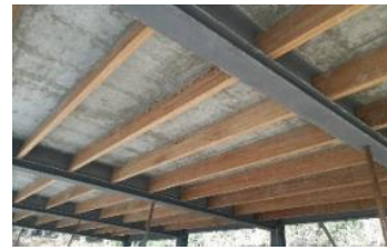
Fig.10. Example of composite glulam and concrete
