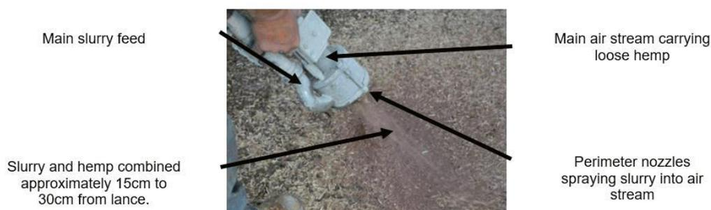
Fig. 1: The projection process and lance.
