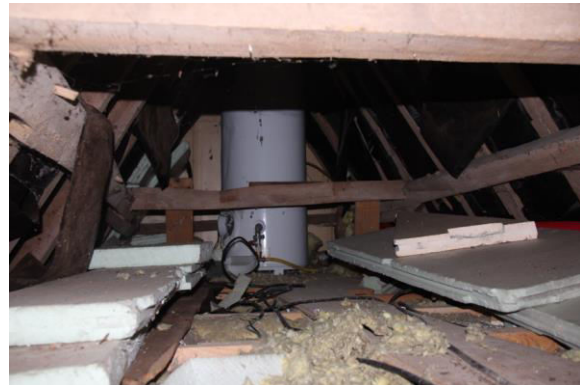
Fig. 9: Attic before thermal rehabilitation (glass wool insulation).
