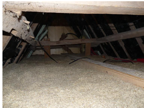
Fig. 10: Attic after thermal rehabilitation with flax shives.
