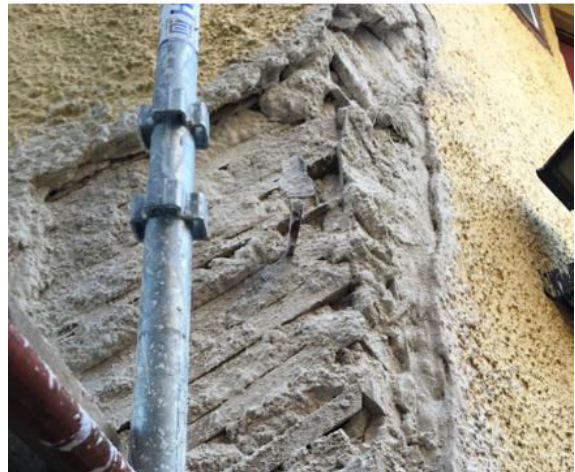
Figure 1. Exposed plaster embedded in wooden slats on a house in Visby. A lime-cement render had been applied in an earlier renovation (yellow render).
