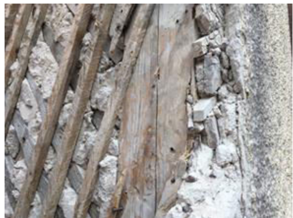
Figure 2. Exposed lime plaster embedded in diagonal wooden slats on another property in Visby. Here the lime and wooden slats were removed in order to apply mineral wool insulation with the goal to improve energy efficiency.
