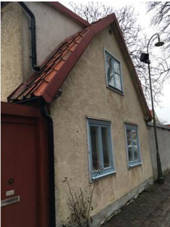
Figure 8. Historical timber building in Visby. The façade will be renovated using lime-hemp in 2017.
