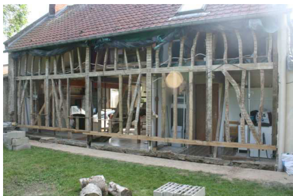
Fig. 6: Wall ready to receive the rape concrete
