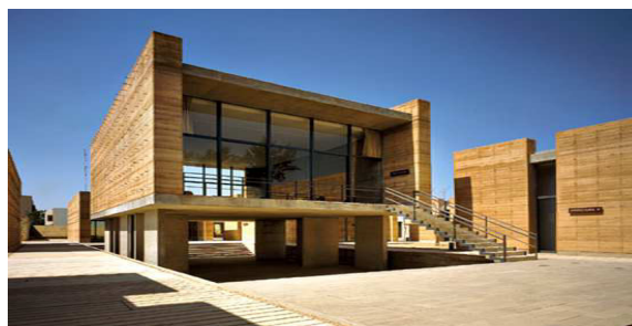
Fig. 3 An example of modern earthen structure: the Oaxaca School of Plastic Arts in Mexico (www.dailytonic.com).
