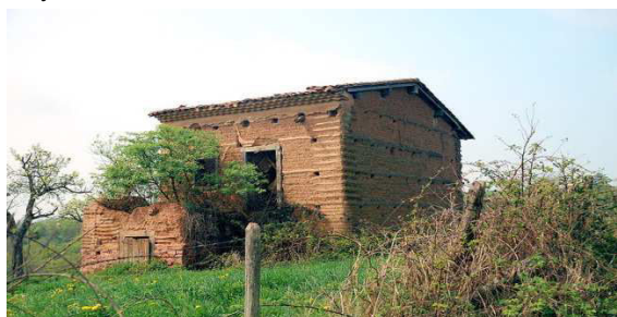
Fig. 2: Traditional house made of rammed earth in Auvergne, France (www.french-property.com).
