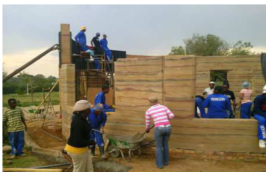
Fig. 1 : Rammed earth construction at Mablomong school(www.specifile.co.za/).
