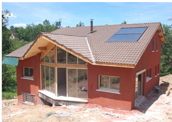
Fig. 1: View of the south façade of the building.
