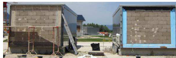
Fig. 1: Passys cells with hempcrete walls
