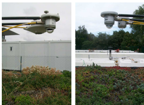
Fig. 3: Pyranometer CMP3 and Pyrgeometer CGR3 used to measure the reflected flux of long and short wave radiation
