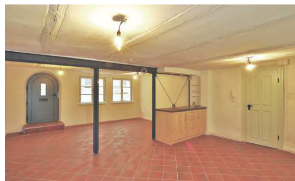
Fig. 14: Photographic view of the room after application of the internal insulation.
