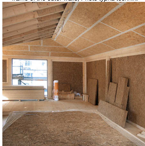
Fig. 21: Internal view of the sauna building under construction; Photo typha technik.
