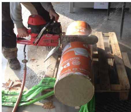
Fig. 5 : Cutting the puddingstone concrete column
