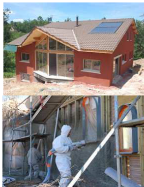
Fig.4: Hempcrete spray application [DB Chanvre photographs]
