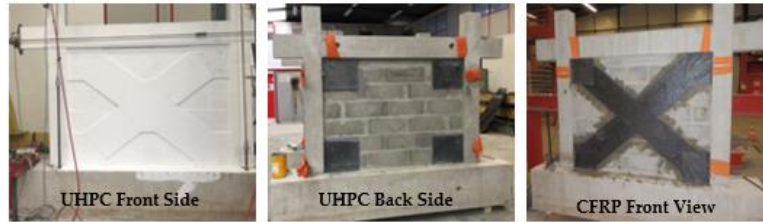
FIGURE 1. Photographical Illustration of Retrofitted Specimens
