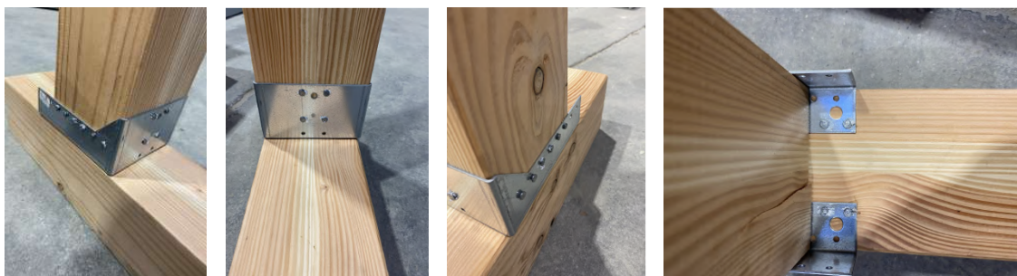
FIGURE 5. Traditional connection (TC): Metal clap (CECOIA 2023) and grooved spikes
