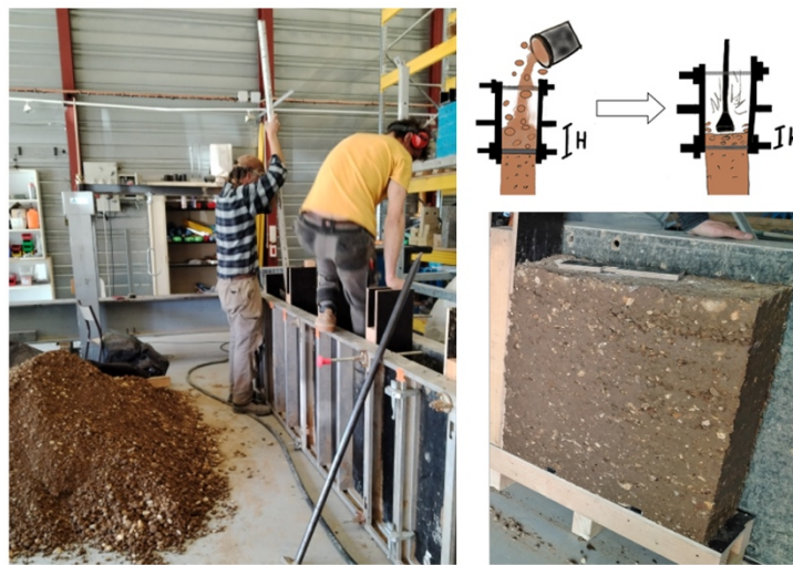
FIGURE 2. Construction of RE wall
