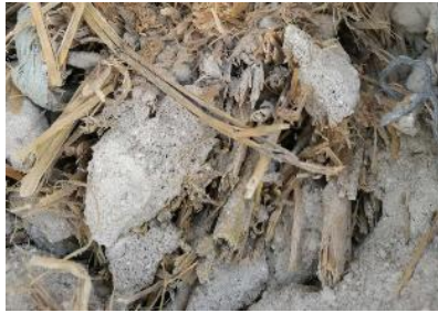
Figure 11. Mixture of straw and lime stucco outside the high position of laid flat bale wall.
