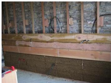
Figure 4: Banchage (200 – 500 kg/m<sup>3</sup>)
