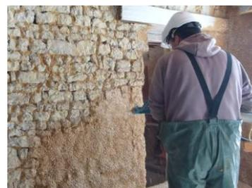
Figure 5: Projection (200 – 500 kg/m<sup>3</sup>)
