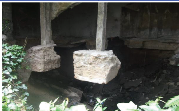
Figure 6. Foundation failure due to Erosion [TCH 16]
