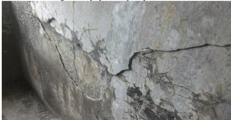
Figure 2. Cracks due to alternating wet / dry cycles (Photo Bonapriso, 2014)
