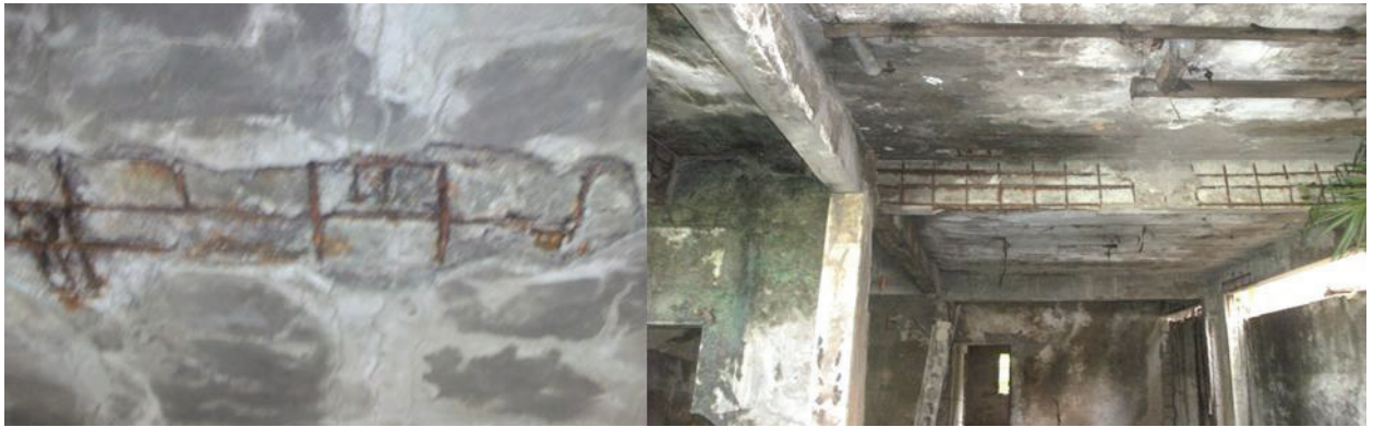
Figure 7. Cracking, spalling, and brownish staining due to corrosion of the reinforcement bars
