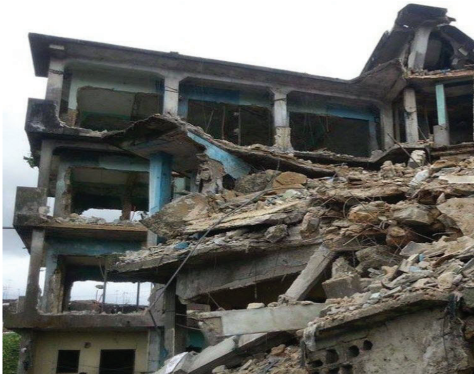
Figure 5. Collapse site of a 4-storey building at Nkoldongo, Yaoundé due to design errors http://fr.africanews.com/2016/06/20/cameroun-cinq-morts-dans-l-effondrement-d-un-immeuble/
